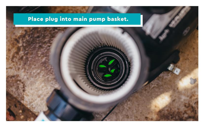
Remove drain plug from your pump and filter. Each pump has 2 drain plugs. After removing, place plugs into main pump basket for safe storage.
