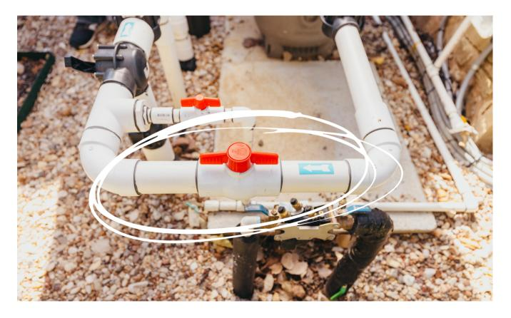
Open all faucet spigots, and undo the air relief on top of the filter.
