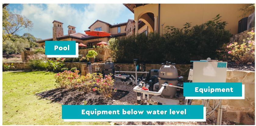
If your pool equipment is below your pool's water level turn all LARGE red ball valves off before removing any drain plugs from your equipment.
